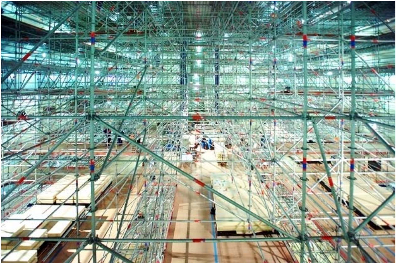
The construction work requires costly scaffolding systems
